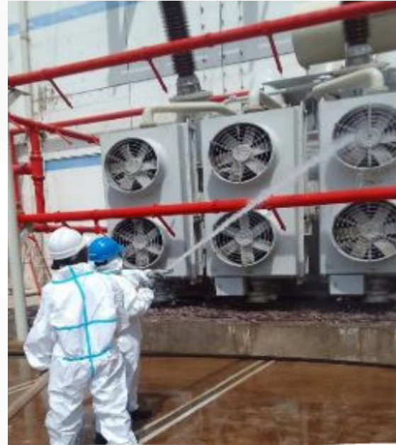
Figure 14: Washing of 54G3 Power Transformer
