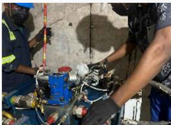
Figure 20: Transferring Oil into the 54T5 Transformer
