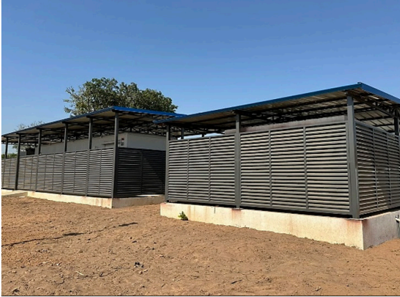
Figure 23: Far left external view of modular datacenter located at BGS
