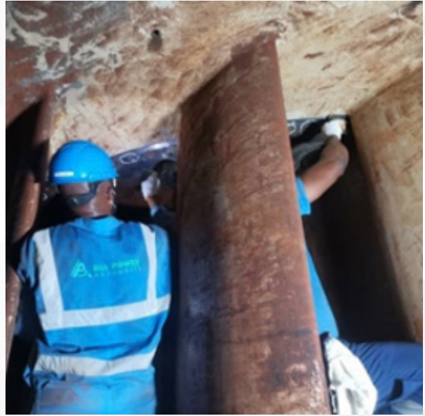
Figure 10: Inserting the stop logs as part of isolation for 54G1 Annual Maintenance
