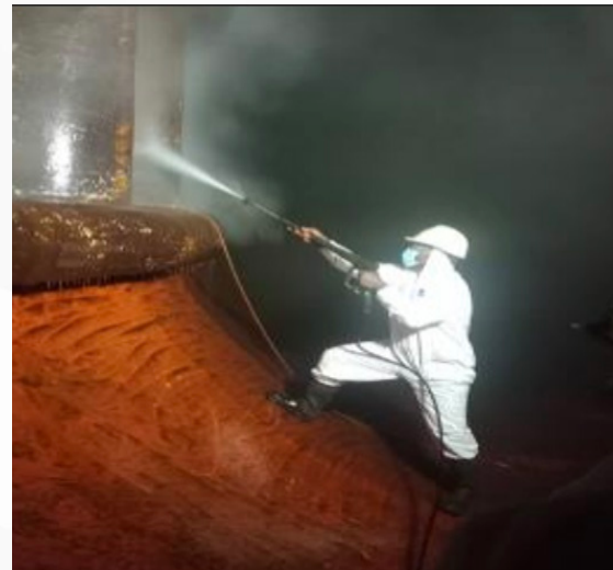
Figure 16: Washing of stay vanes in spiral case
