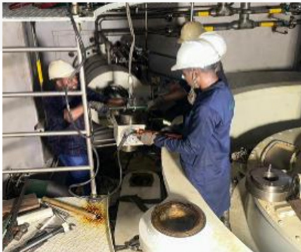
Figure 15: Replacement of defective Seals in the Servomotor
