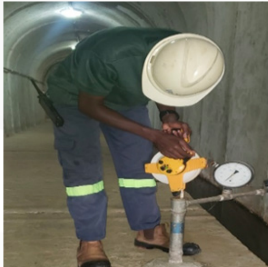
Figure 8a: Measurement of seepage in dam body
