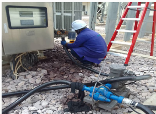
Figure 19: Cleaning and inspection of 54G5 intake hydraulic unit
