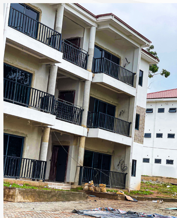
Figure 21: Staff Accommodation Project
