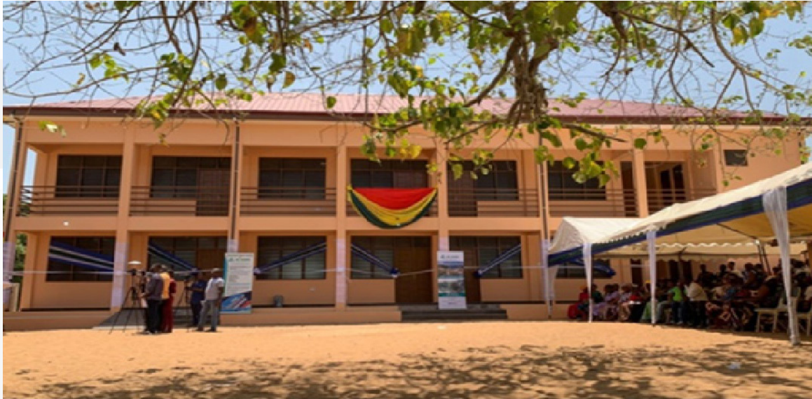
Figure 28: Front view of Six-unit classroom block
