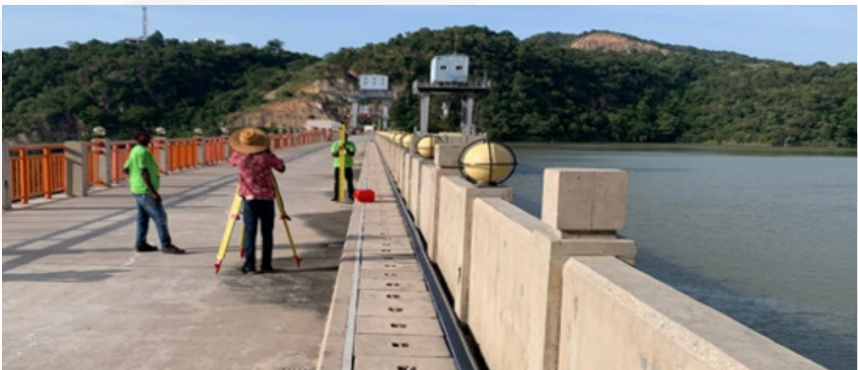
Figure 7: Deformation monitoring survey activity
