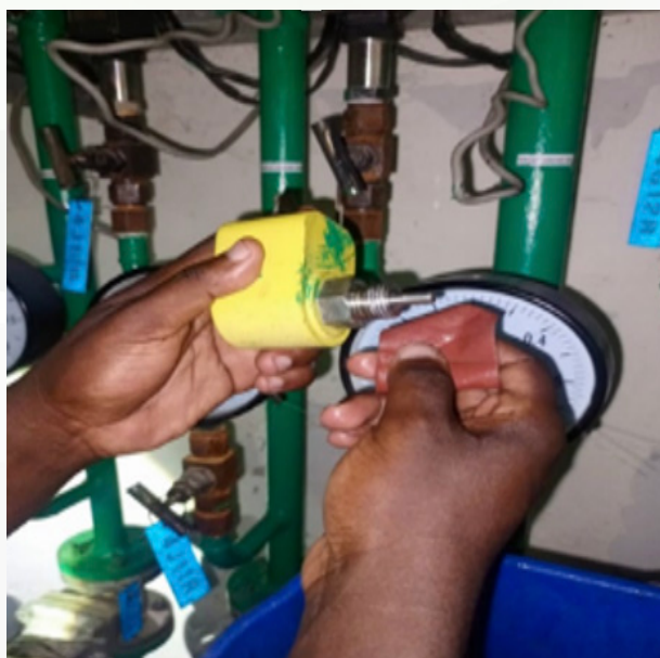
Figure 17: Pictures from 54G4 Annual Maintenance Activities
